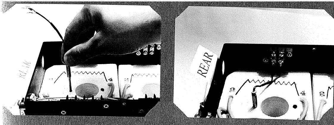
FIGURE 2: Installation of TC in well and wiring to Terminal strip.
